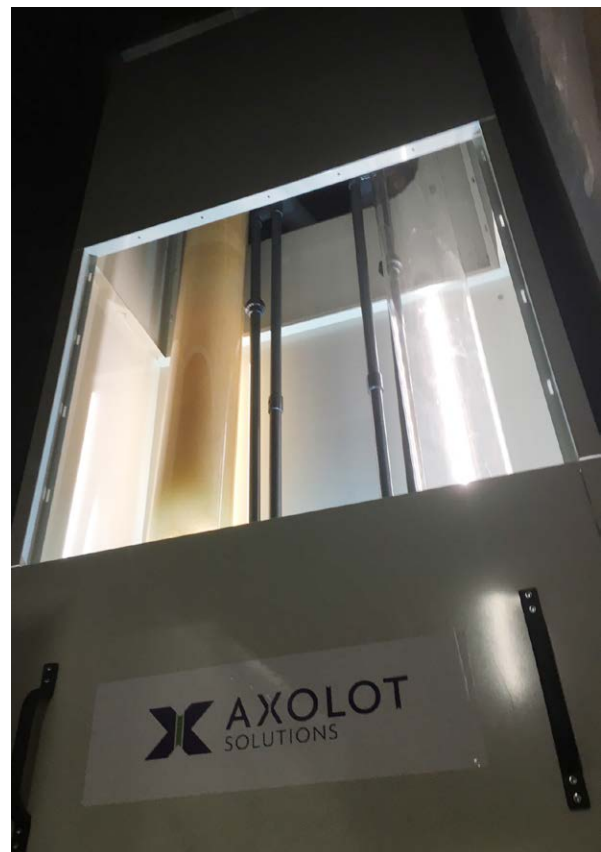
Axolot's first wastewater purification unit has successfully been started up during the first quarter.
